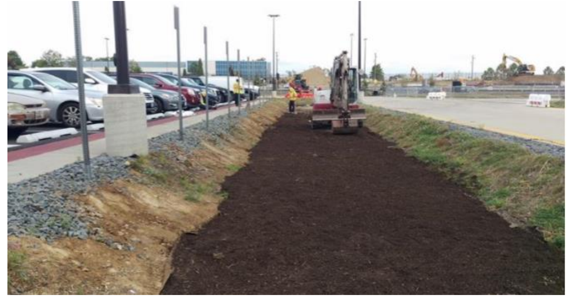
Grading in Bio Pond Water Quality Structure
