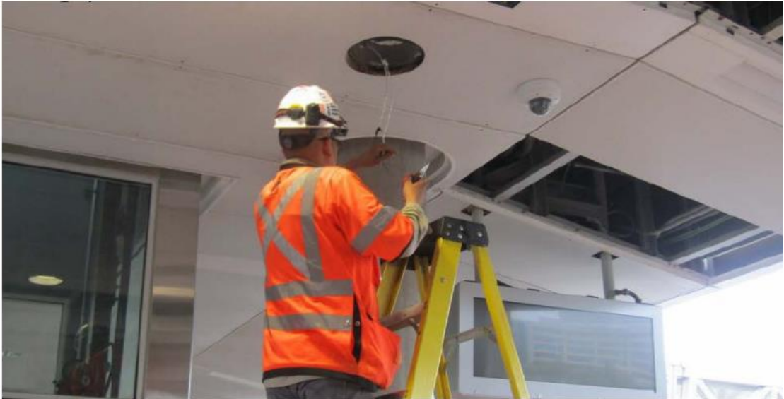
Installing Speakers in Ceiling Panels at Reston Station
